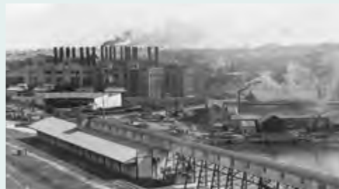
View of Balmain Power Station and White Bay headwaters from Glebe Island grain silos, c1940s.
