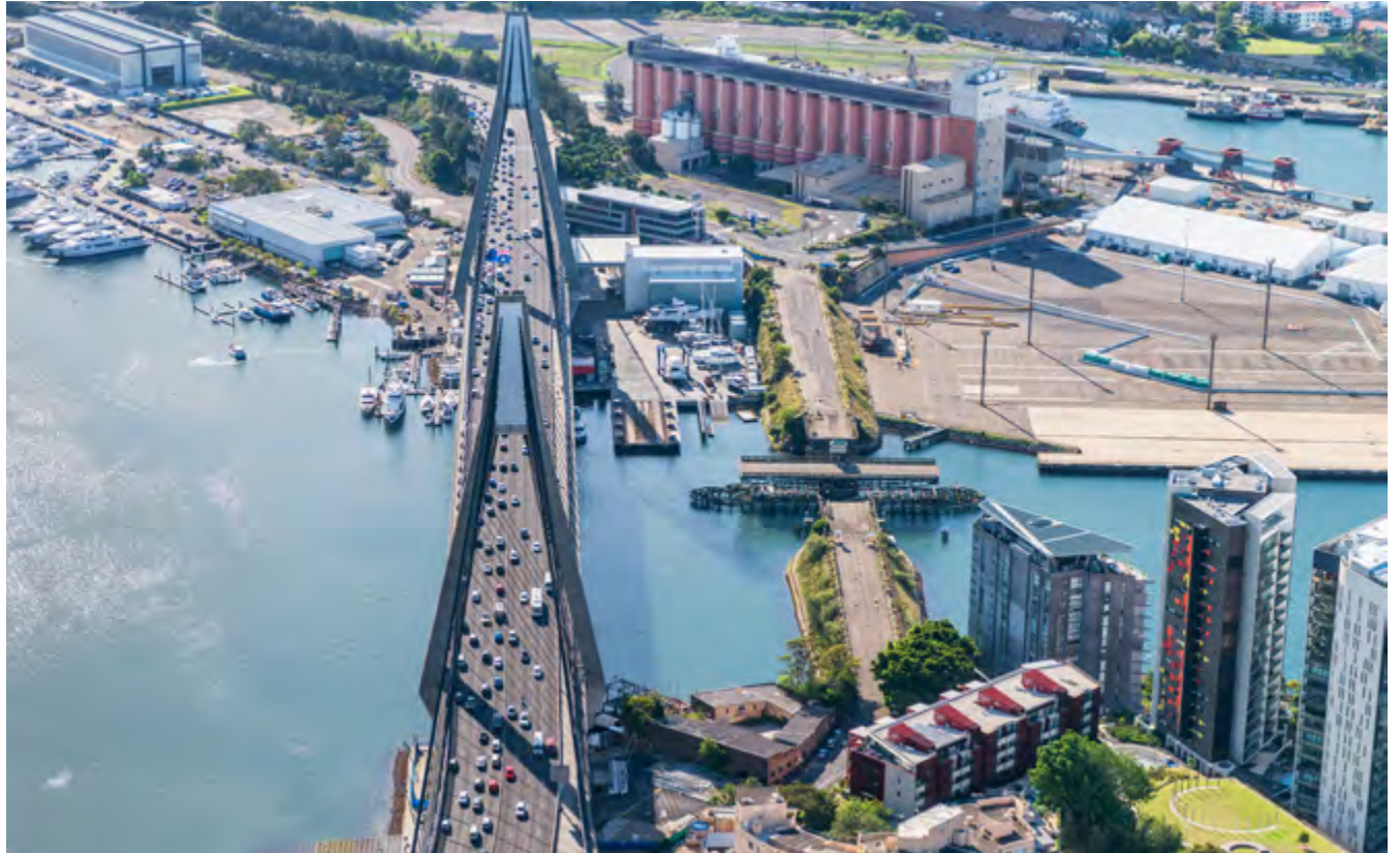
ANZAC Bridge shown on the left and Glebe Island Bridge on the right.
