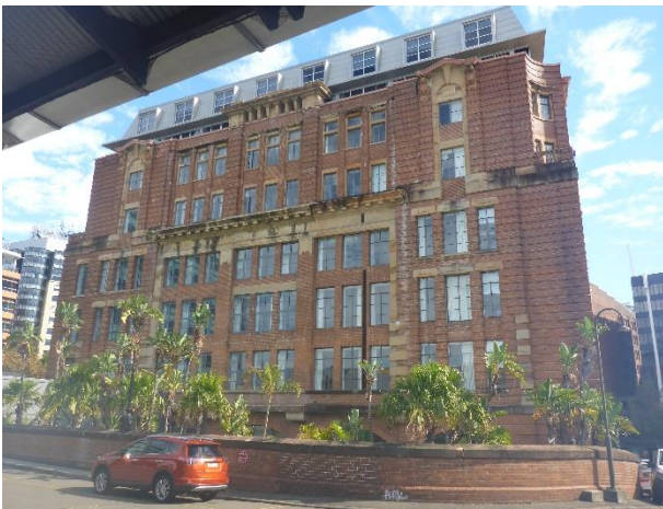
Figure 36 – East elevation as viewed from the YHA Railway Square. Note the brick retaining wall that defines the rear yard.
