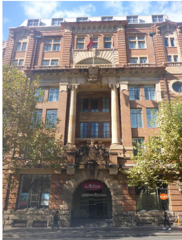
Figure 31 – Primary (west) elevation of the site as viewed from Railway Square
