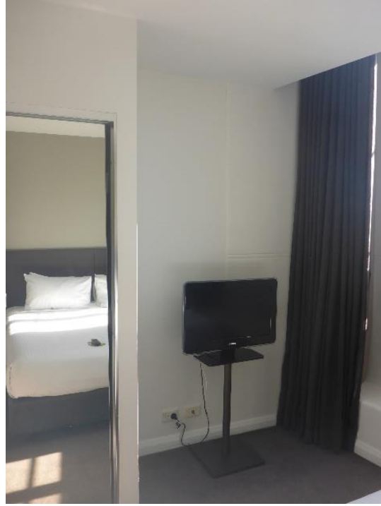
Figure 77 – Bedroom wall. Note the interface with the original structure and the later partition Source: Urbis, 2019Urbis, 2019
