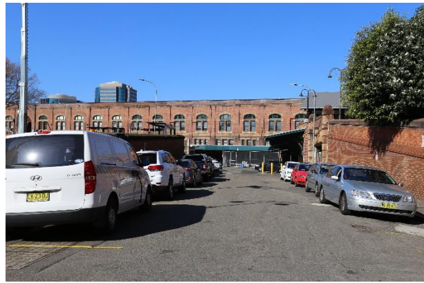
Figure 26 – View towards central station and the vehicle access to the rear yard of the parcels post building, and showing the ramp to the Inwards Parcels building on the far right
