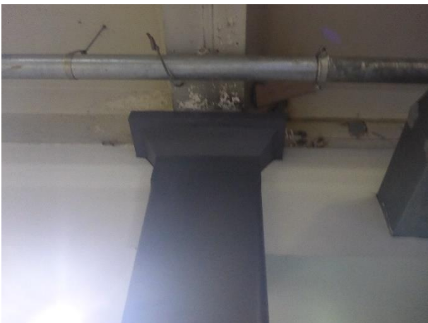
Figure 104 – Exposed column capital
