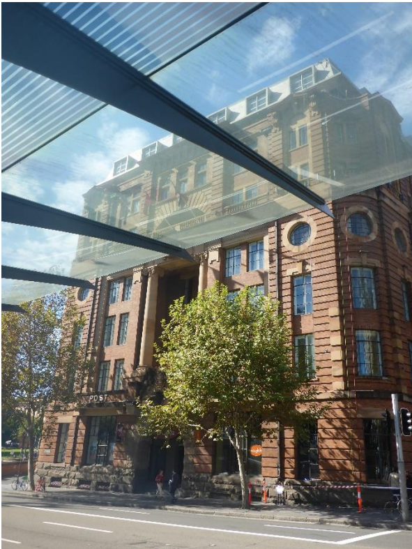
Figure 30 – Primary (west) elevation of the site as viewed from Railway Square
