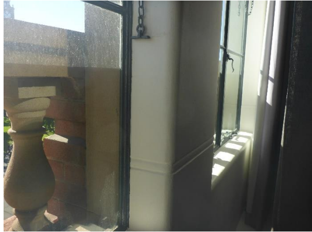
Figure 71 – Detail of the steel framed windows, wall detail (dado) and external sandstone detail (baluster) Source: Urbis, 2019Urbis, 2019
