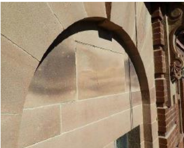
Figure 122 – Delamination on stone
