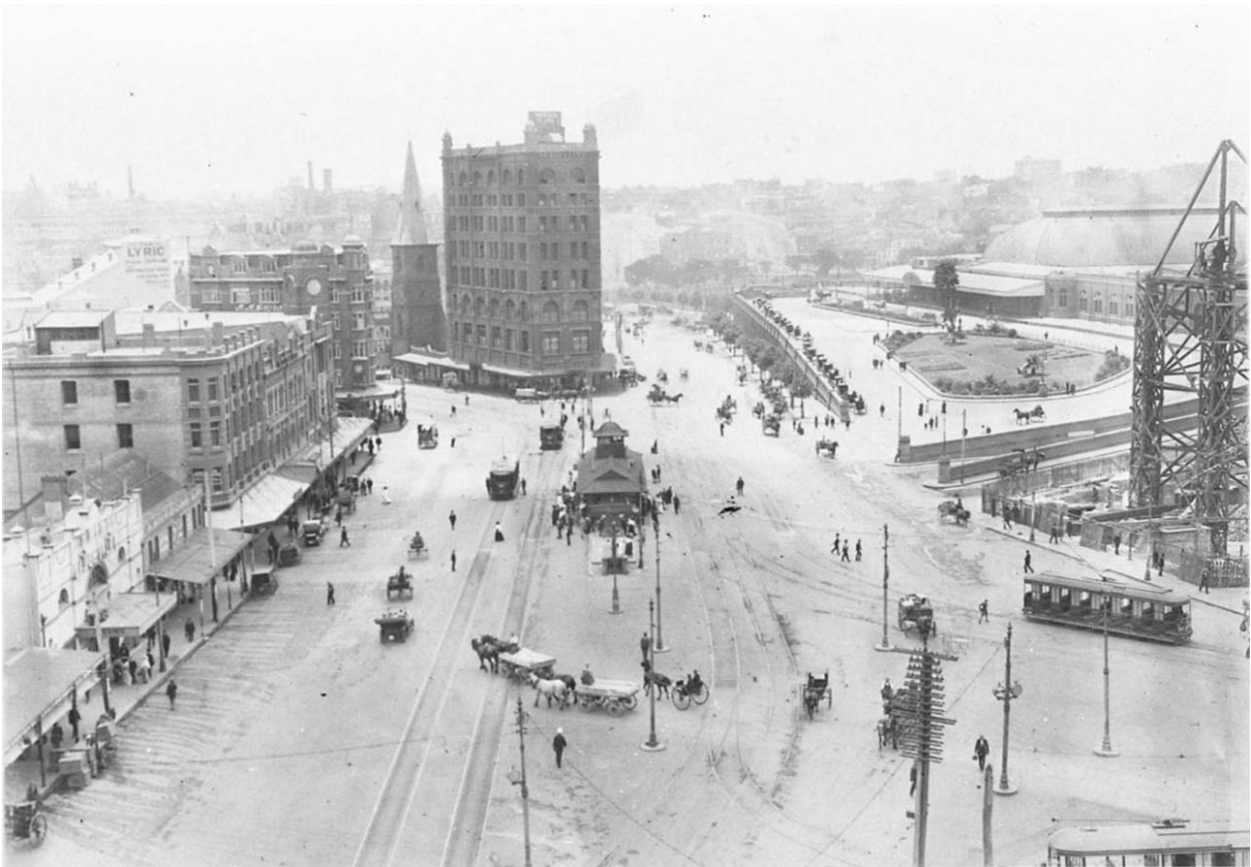
Figure 135 – Railway Square before the Central Railway clock tower was built, 1911. In this view (at far right) scaffolding and gantry on site of future Parcels Post Office building.
