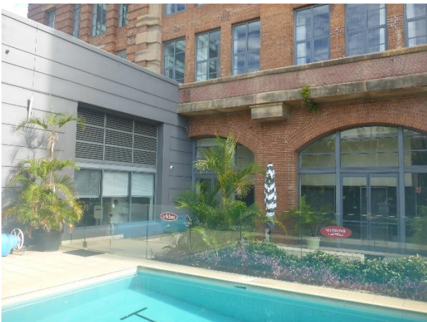
Figure 100 – The contemporary addition and interface with the former vehicle dock opening
