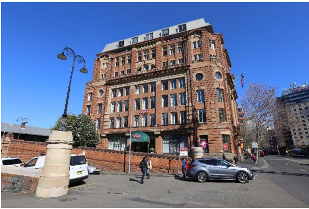
Figure 25 – The northern façade of the subject Parcels Post building and the ramp/ vehicle access to upper level of the neighbouring Inwards Parcels building
