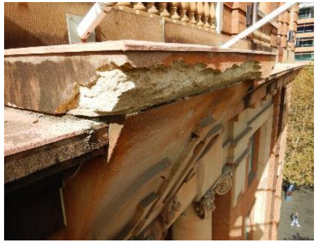
Figure 119 – Sandstone embellishment after removal
