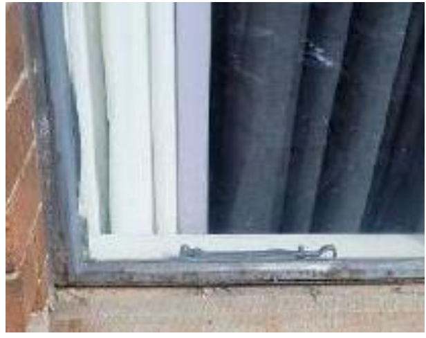
Figure 121 – Typical condition of steel windows
