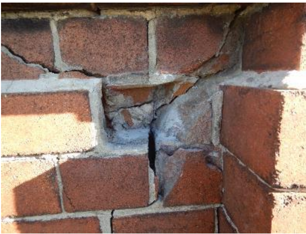
Figure 116 – Broken Bricks
