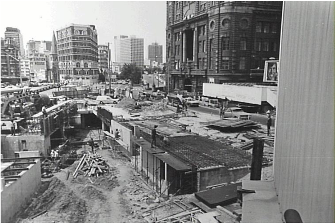
Figure 166 – Devonshire Tunnel construction, Railway Square, 1974
