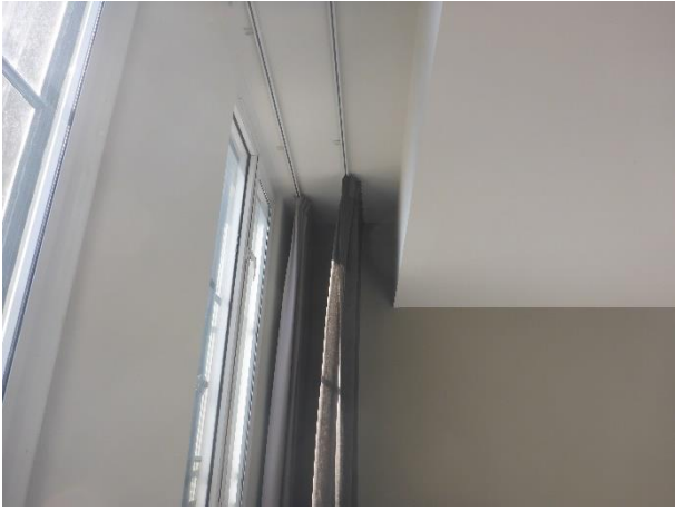
Figure 80 – Detailed view of dropped ceiling and window Source: Urbis, 2019Urbis, 2019
