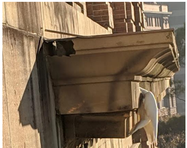
Figure 123 – Styrofoam precast being eaten by cockatoos
