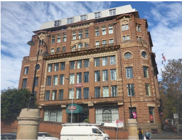
Figure 34 – North elevation of subject building as viewed from Ambulance Avenue. Note the sandstone piers and brick wall defining the level changes and ramps
