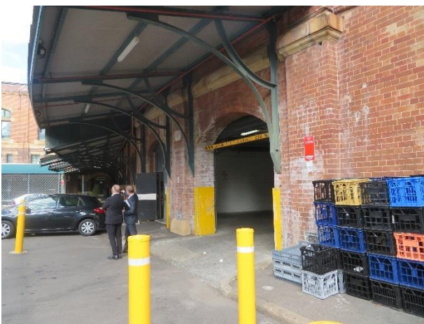
Figure 27 – Lower ground level of the former Parcels area – off Ambulance Lane
