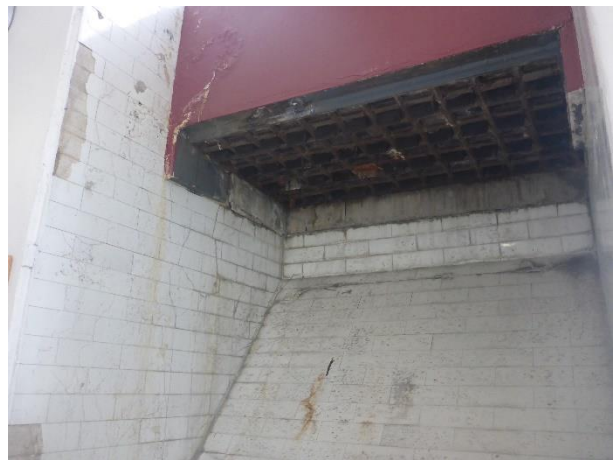
Figure 109 – Tiled over pavement light Source: Urbis, 2019Urbis, 2019
