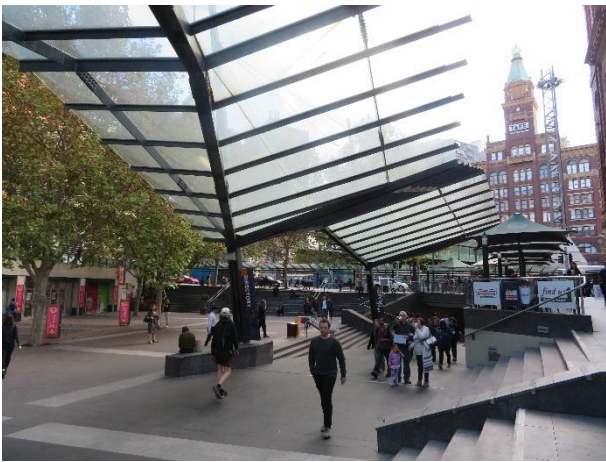
Figure 17 – View of Henry Deane Plaza from the entry to the Devonshire Street tunnel
