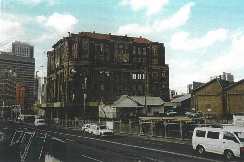
Figure 168 – Subject building and Henry Deane Plaza, c. 1993. Note deteriorated condition of subject building, intrusive awning (since removed).
