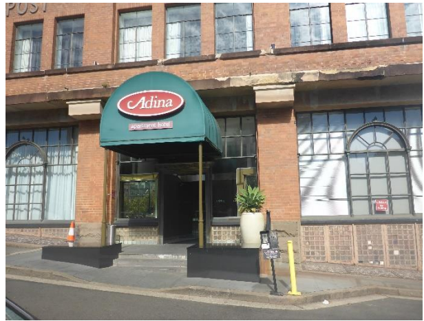
Figure 35 – Awning and accessible entrance of the north elevation. Note the extant stallboard and pavement lights.
