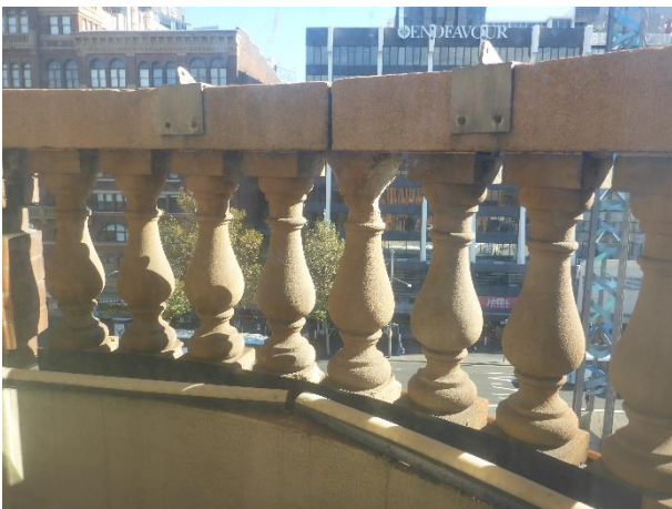
Figure 82 – Sandstone façade balusters Source: Urbis, 2019Urbis, 2019
