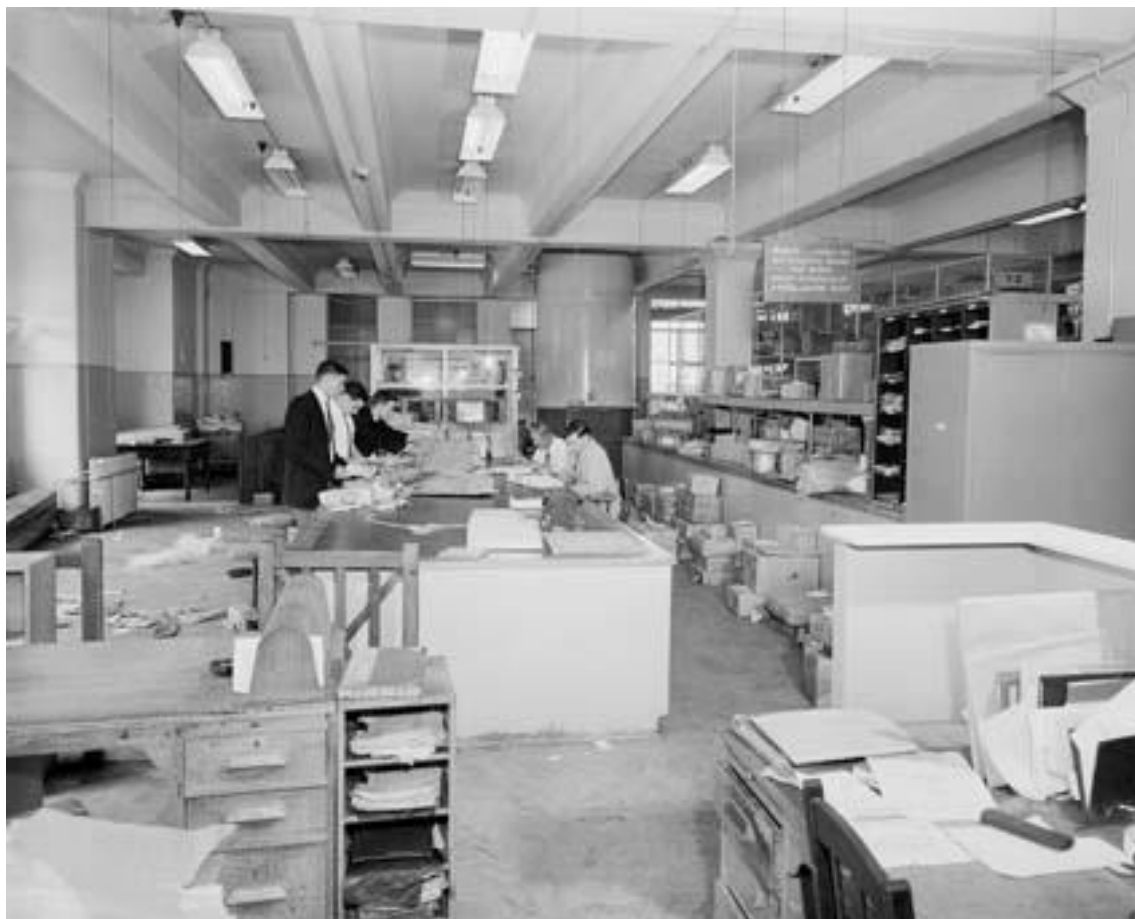
Figure 164 – Working conditions in Chief Parcels Office, Central Square, 1960.
