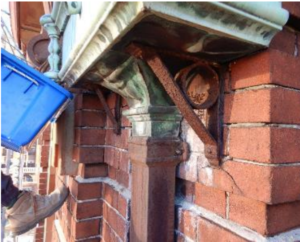
Figure 120 – Corroded steel fixing
