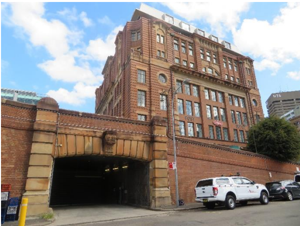
Figure 102 – Vehicle entry to the basement level. Note the ornate sandstone framing.
