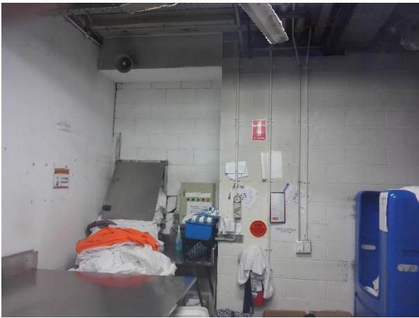
Figure 106 – Basement view Source: Urbis, 2019Urbis, 2019
