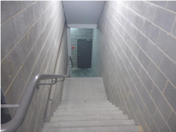
Figure 94 – View of staircase to plant room
