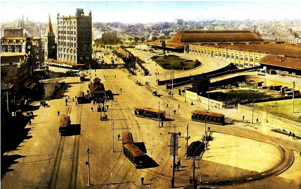
Figure 125 – Railway Square, c.1906-1911. Site of future Parcels Post Office shown in this view as vacant land with hoarding to George Street frontage (centre right).
