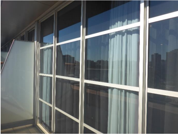
Figure 46 – Façade glazing to the c.1999 mansard addition
