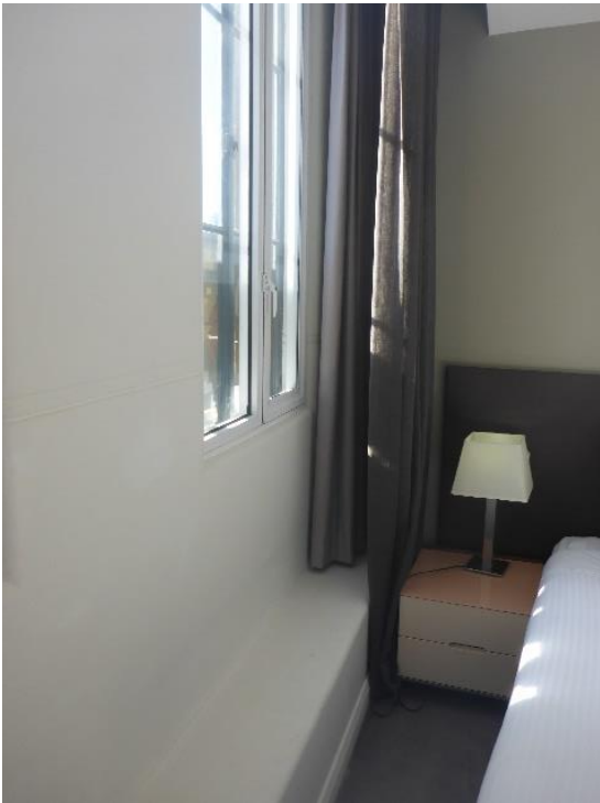
Figure 78 – Detail of the inner face of the external wall Source: Urbis, 2019Urbis, 2019
