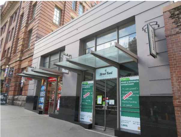
Figure 44 – Contemporary addition on south elevation. This element operates as retail tenancies to the south (as shown) and as the gym for Adina Central to the north.
