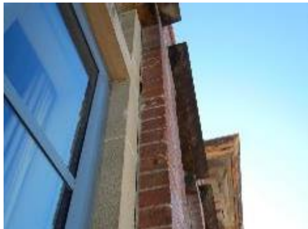
Figure 117 – Stack bonded cladding with no ties
