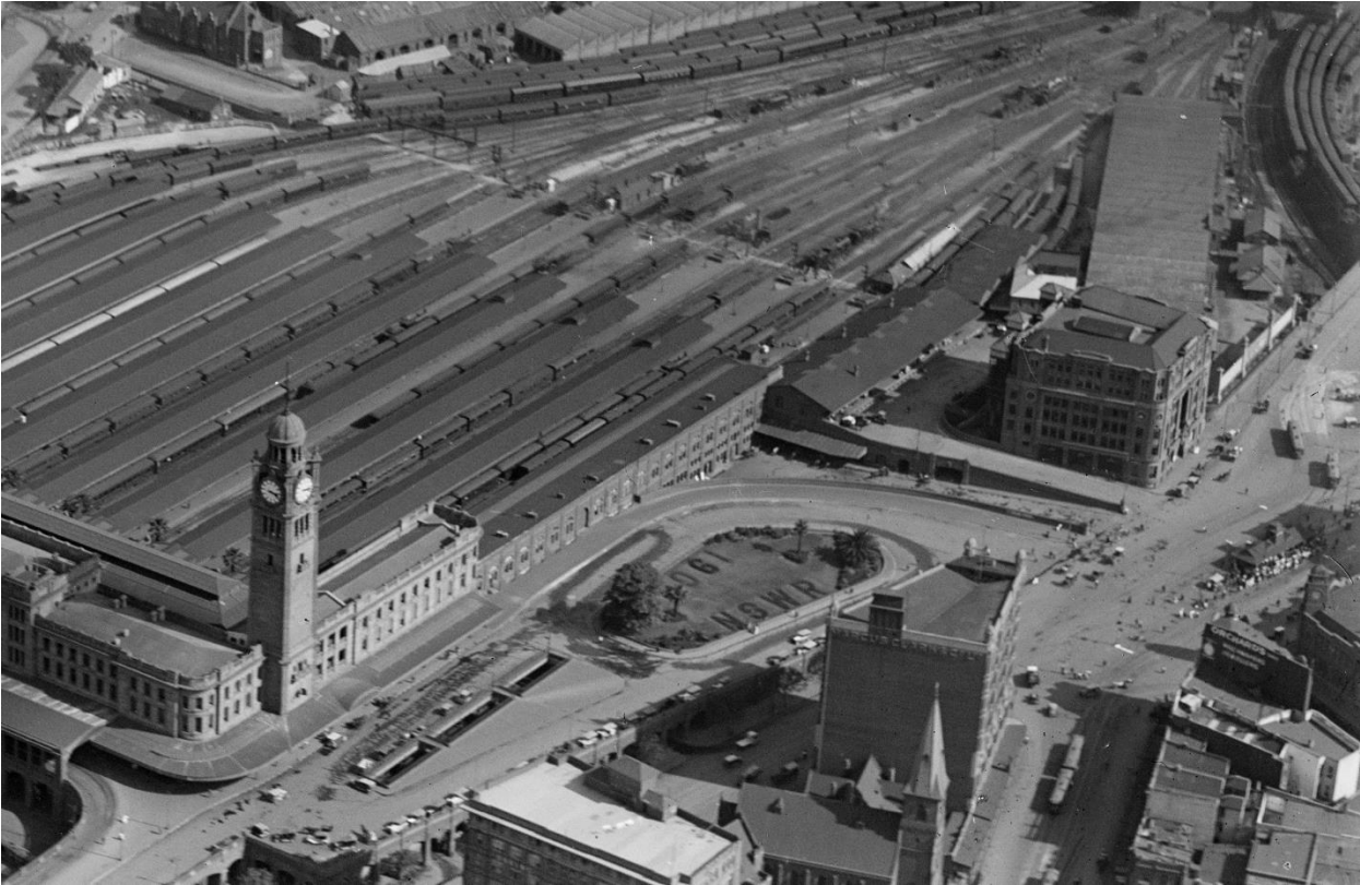
Figure 150 – Aerial of locality c. 1920-1938. Note the relationship between the subject site and former Inwards Parcels Shed (now YHA Railway Square), Central Station, and Western Forecourt.
