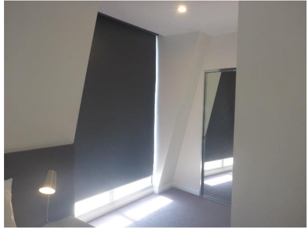
Figure 91 – View of window in mansard addition
