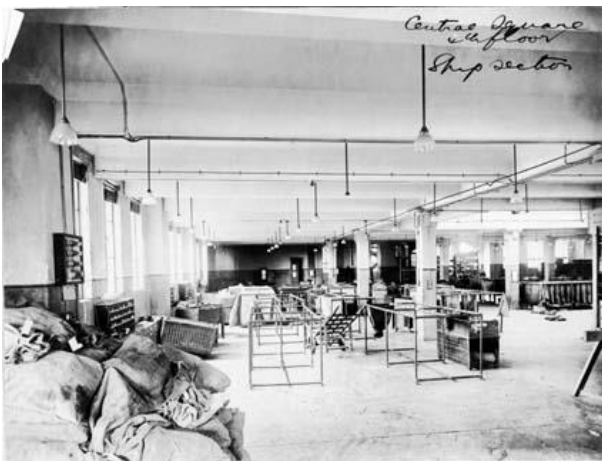
Figure 142 – Fourth floor (ship section), Central Square Building, c.1910s.
