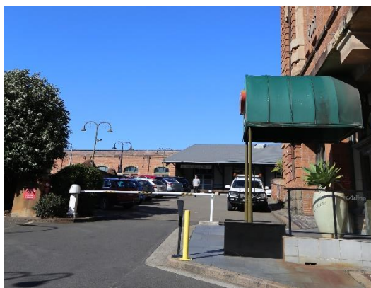
Figure 23 – View east towards the Inwards Parcels shed from Lee Street with the Parcels Post at right
