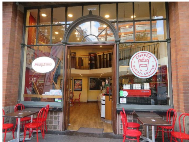
Figure 43 – Shopfront on south elevation. Note the extant stallboard lights and intact fenestration
