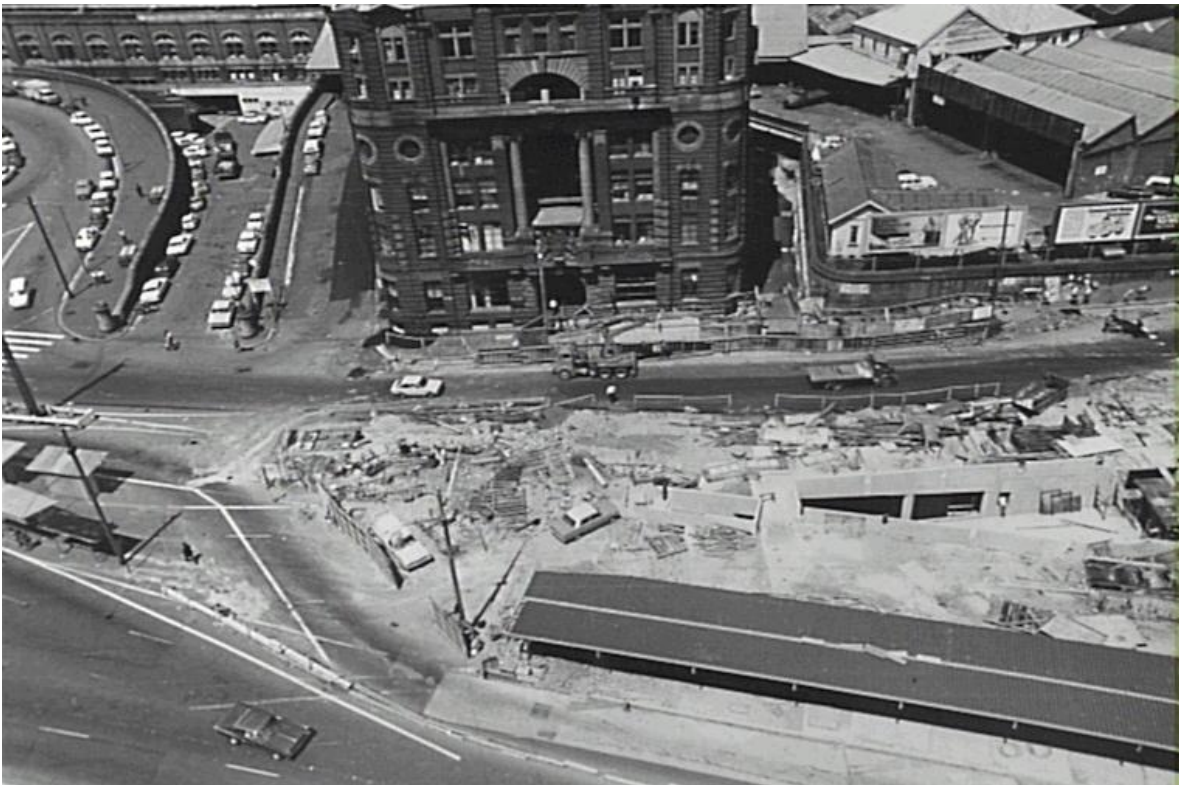
Figure 167 – Devonshire Tunnel construction, Railway Square, 1975
