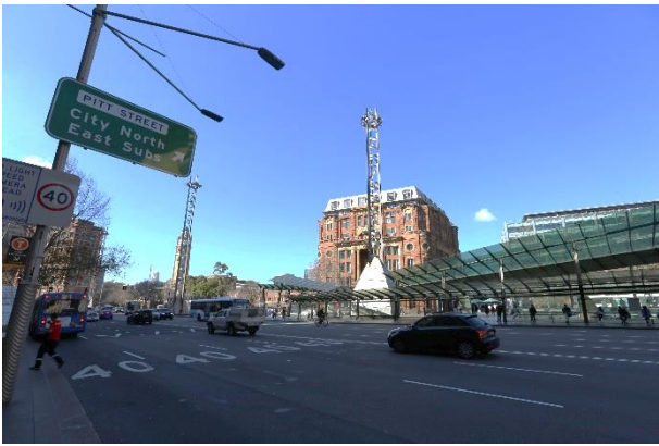
Figure 28 – Glass awnings of Railway Square Source: Urbis, 2019Urbis, 2019
