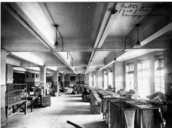
Figure 140 – Second floor (newspaper sorting), Central Square Building, c.1910s.
