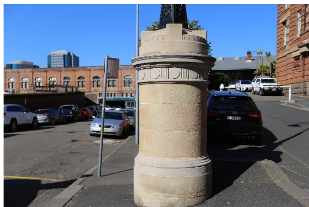
Figure 24 – Sandstone element marking the entrance to the YHA Railway Square
