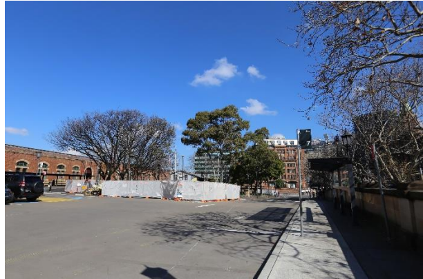
Figure 12 – Western Forecourt facing south, central landscaped element obstructed by barricade
