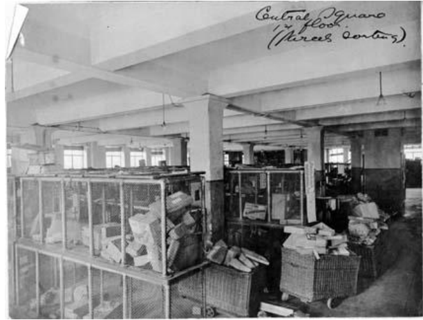
Figure 139 – First floor, Central Square Building, c.1910s.
