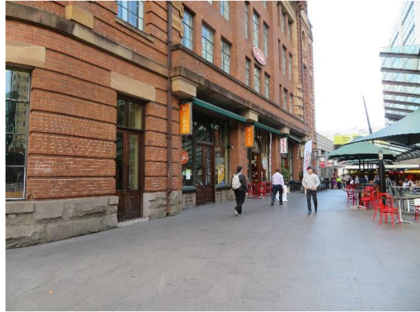
Figure 41 – Shopfronts on south elevation.
