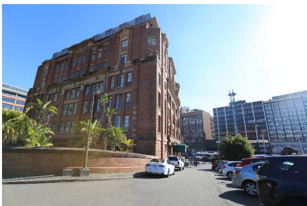
Figure 21 – View west towards Lee Street from the forecourt of the Inwards Parcels shed
