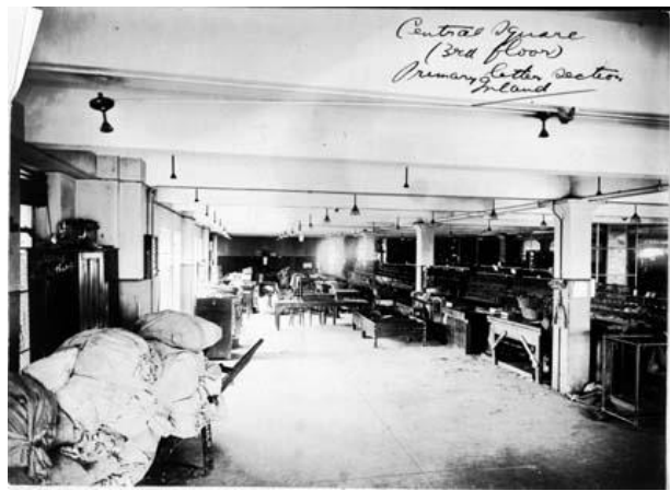
Figure 141 – Third floor (primary letter section inland) Central Square Building, c.1910s.
