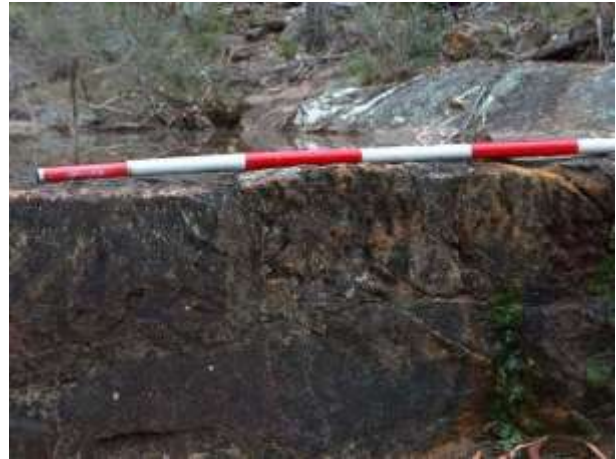
Plate 2: View facing south of sandstone weir crossing Allens Creek. Note the sandstone hammer dressed blocks display sparrow picking
