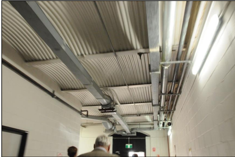
Figure 36: The Basement area storeroom. Note corrugated iron formwork forming an arch to support the structure above.
