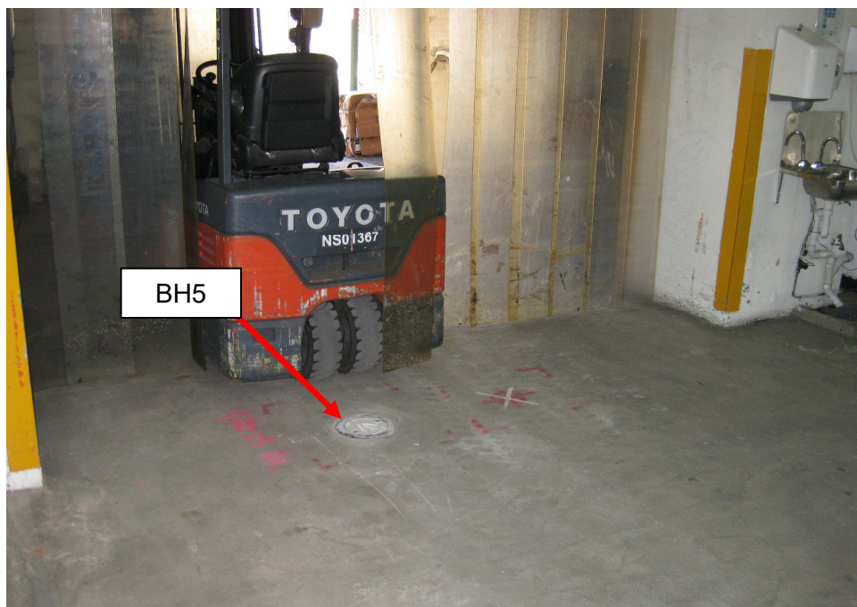
Photo 14 – View to the north-east at the location of Borehole BH5, indicated as shown. A metal lid covers the hole, below which a standpipe piezometer has been installed.
