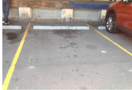
View of: Oil staining on bitumen car park area Looking: East
