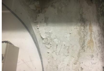
View of : Flaking paint within underground service tunnels. May contain Lead. Inspected on 24.11.2017
