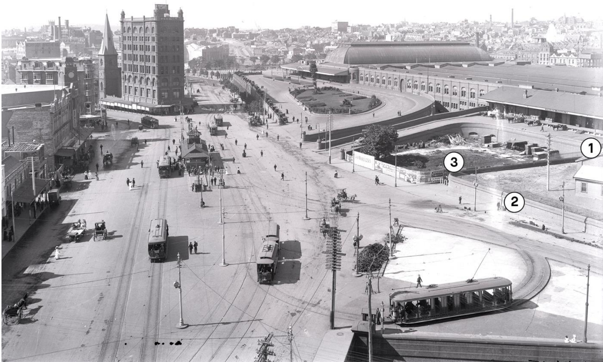
Figure 3.11 1908 view to the northeast across the newly constructed Central Station. The entrance to the Devonshire Street tunnel is shown at (1). The Site (2) is partially visible at the right-hand side—its retaining wall indicates the depth of fill imported to raise the site above street level. (3) is the site of the Parcels Post Office under construction. (Source: NSW State Archives and Records Authority 1740 a014 a014001399 with GML additions)
