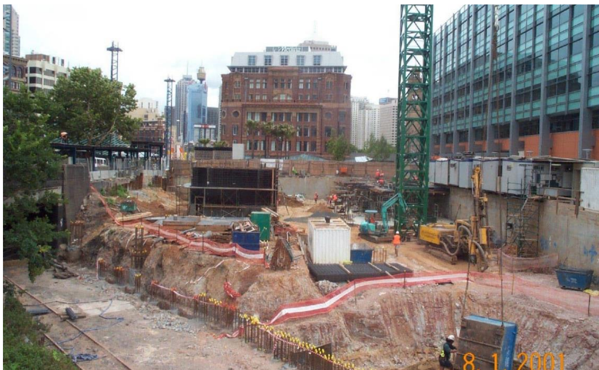
Figure 2.12 Northern view of part of the Site showing the ground level excavated to bedrock. The Goods Line can be seen in the foreground. (Source: Frasers)
