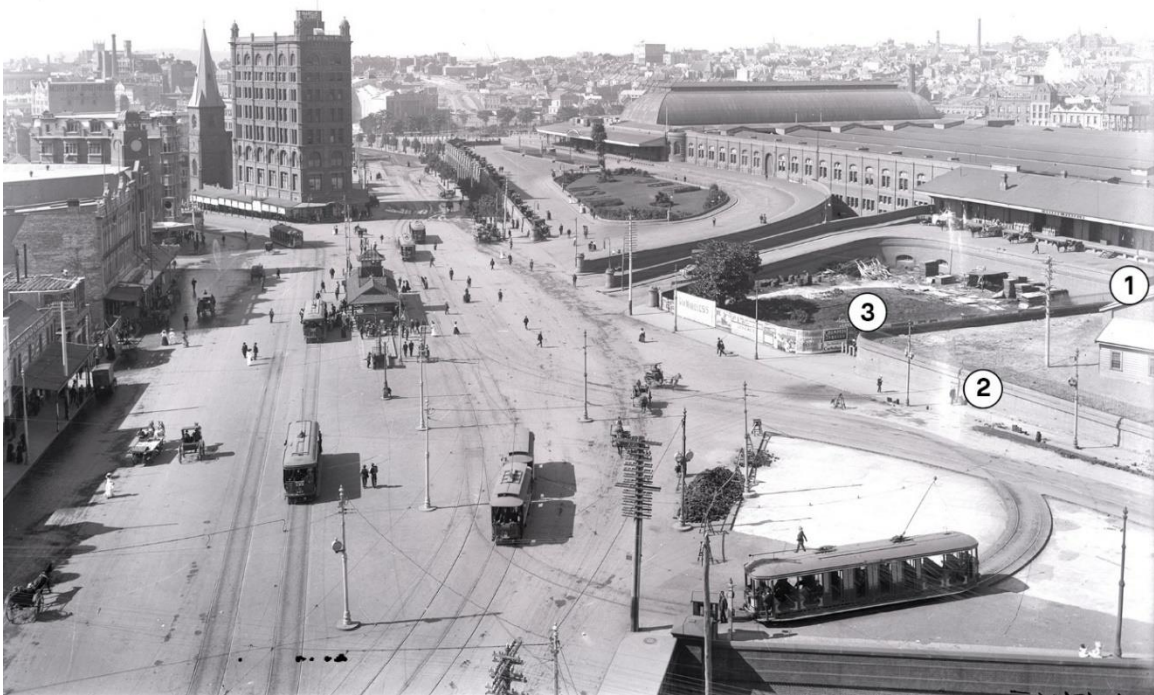
Figure 2.8 1908 view to the northeast across the newly constructed Central Station. The entrance to the Devonshire Street tunnel is shown at (1). The Site (2) is partially visible at the right-hand side—its retaining wall indicates the depth of fill imported to raise the site above street level. (3) is the site of the Parcels Post Office under construction. (Source: NSW State Archives and Records Authority 1740 a014 a014001399 with GML additions)
