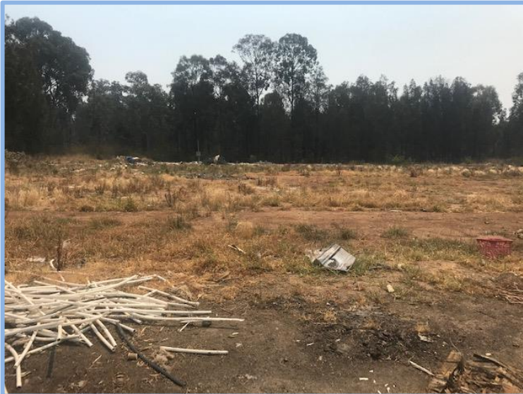
Photo 6-View facing north across cleared portion of site identified for Drainage basin
