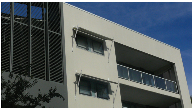
Figure 26. Horizontal sun shading over west facing windows from undesirable heat gain
