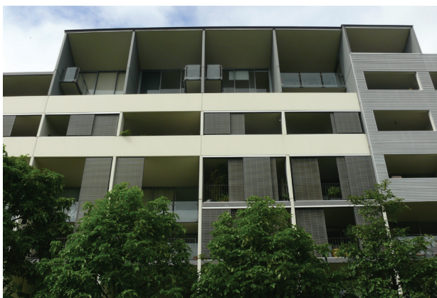
Figure 27. Deep balconies and adjustable screen shade windows from undesirable heat gain
