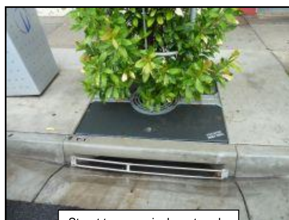
Street tree passively watered from stormwater runoff
