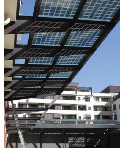
Figure 8C.1-3: Photovoltaic cells integrated into the awning design.
