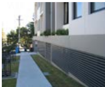
Figure 22.3-2: Ventilation grilles to basement car park are well integrated with overall facade design.
