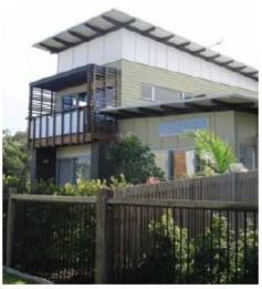
Articulated front elevation with light weight material to upper level and good eaves extension, sun shades / screens used to breakup facade
