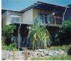
Articulated front elevation with light weight material to upper level and good eaves extention, sun shades / screens used to breakup facade
