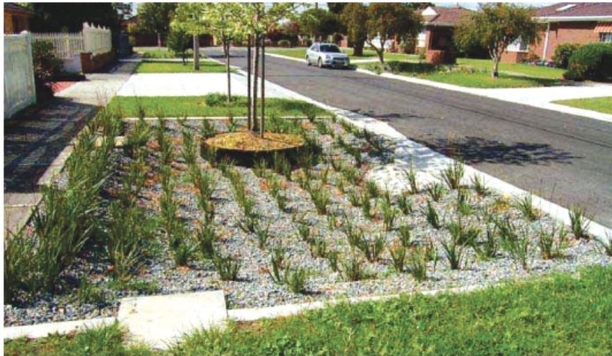
Figure 106: Example of typical bioretention system along roadway
