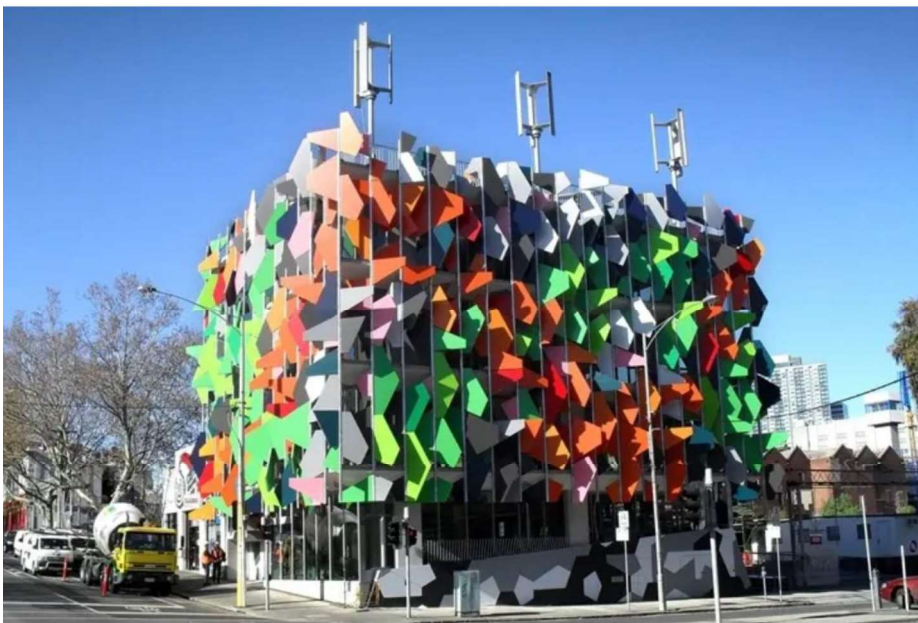
Figure 11: Pixel Office Building by Studio 505, Australia’s first NZEB office building
