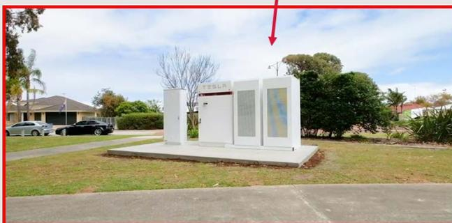
Western Power is currently trialling a 105kW (420kWh) electricity storage system, known as PowerBank, in Meadow Springs, Western Australia. The battery draws power from 52 residential solar energy systems.
