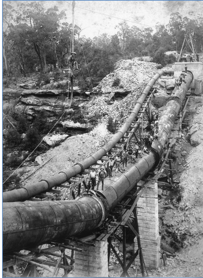
Figure 24 - Leafy Creek Aqueduct sometime between 1886 and 1888 showing the temporary Hudson's scheme aqueduct
