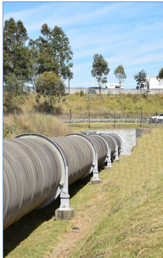
Figure 3 - The Warragamba Pipelines extending underground to run under a road
