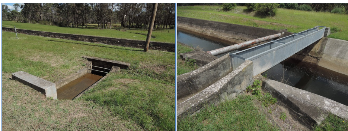
Figure 20 – Examples of Upper Canal drainage systems (left – culvert, right – steel box flume)
