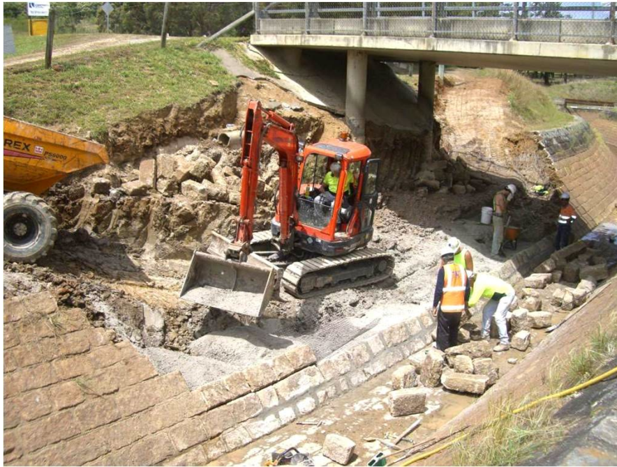
Figure 19 - Reconstruction of Upper Canal wall collapse (2008)
