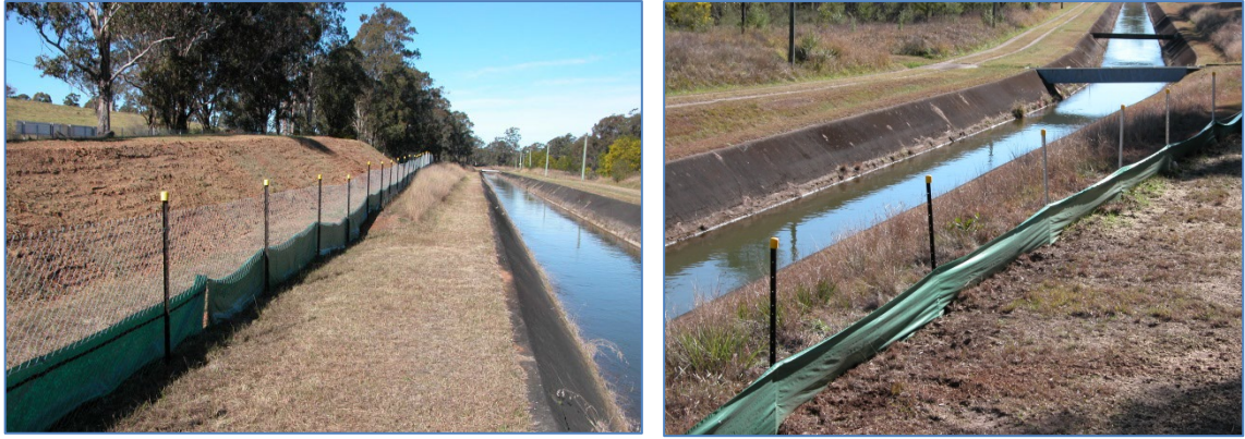
Figure 21 - Erosion control at works adjacent to the Upper Canal
