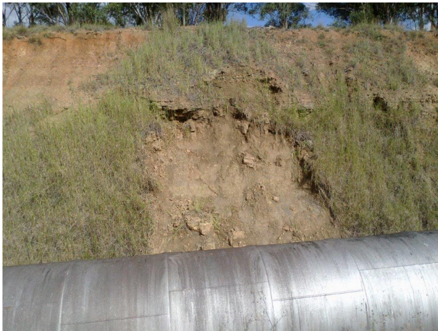
Figure 18 - Embankment slippage along the Warragamba Pipelines Corridor
