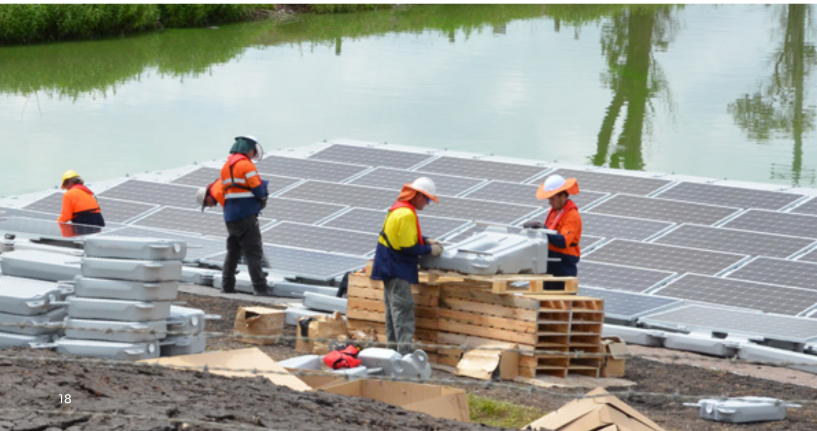
▼ Left-Right: Installation of floating solar panels, Lismore
