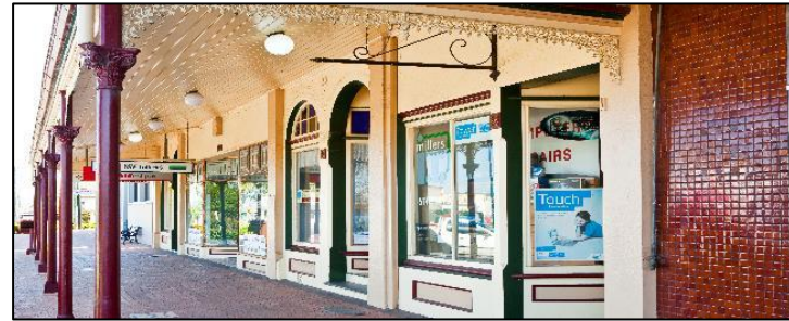
Figure 17 - Commercial heritage buildings in Quirindi.
