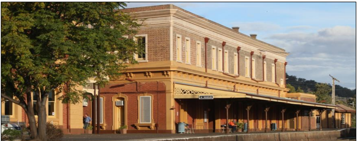
Figure 18 - Werris Creek Railway Station.
