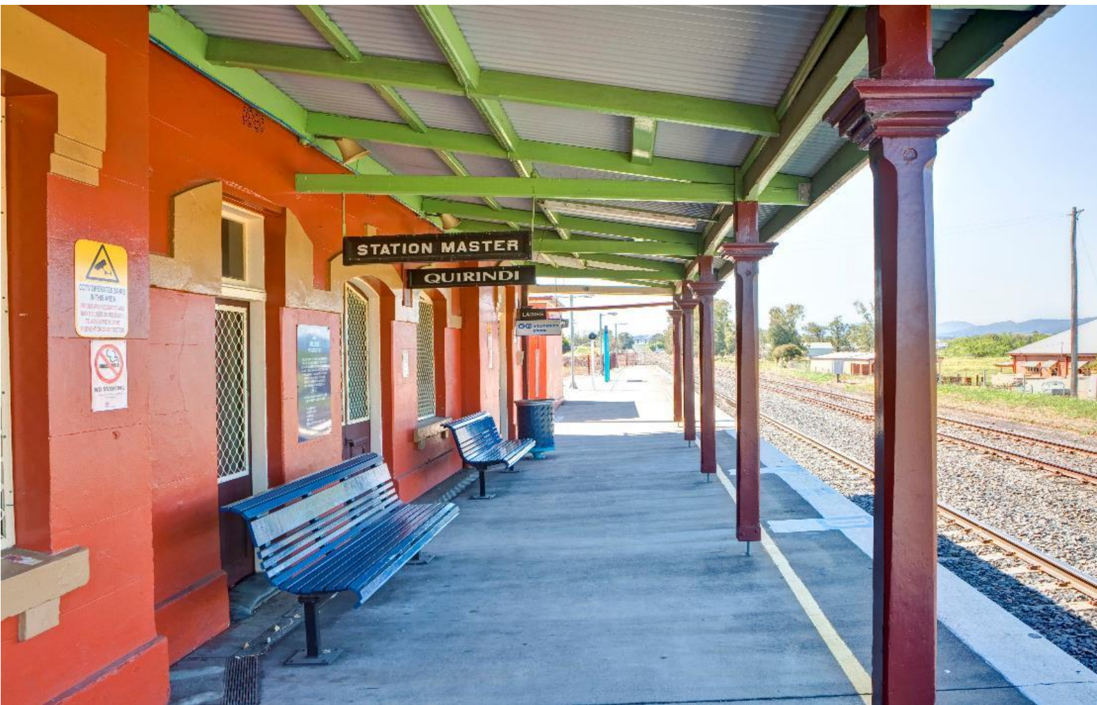
Figure 16 - Quirindi Railway Station.
