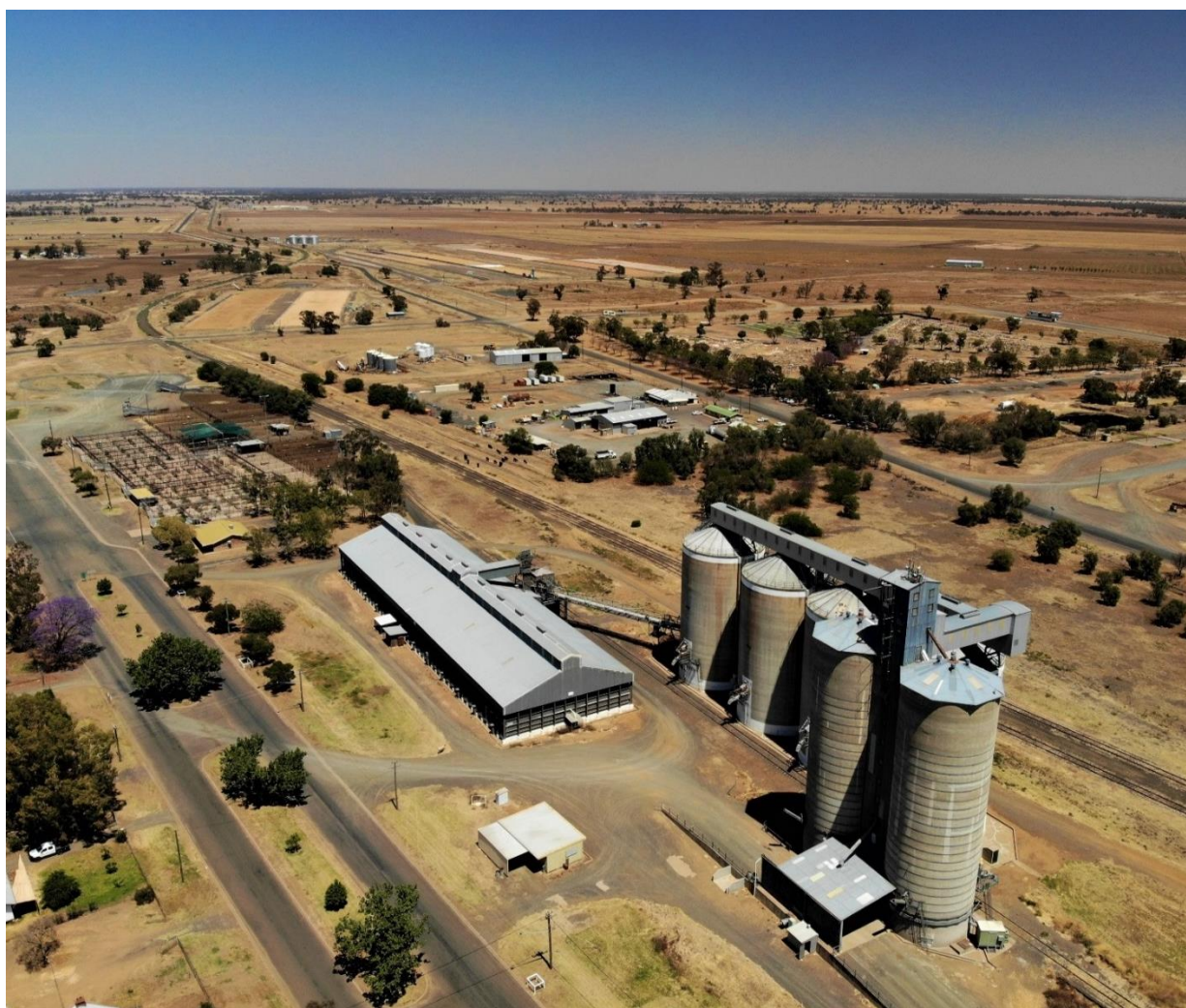
Figure 13 Coonamble Saleyards and railway-side grain storage
