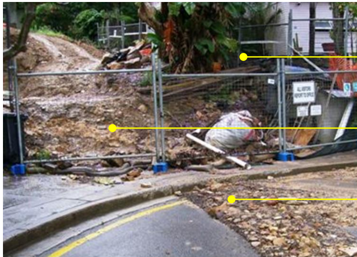
Inadequate erosion and sediment control measures
