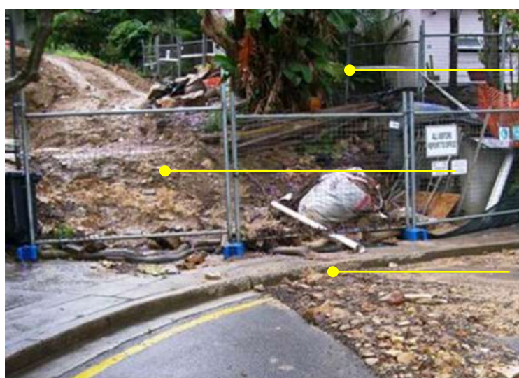
Inadequate erosion and sediment control measures
