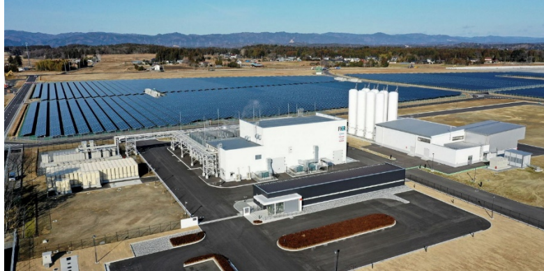
Figure 35: Fukushima Green Hydrogen Plant
