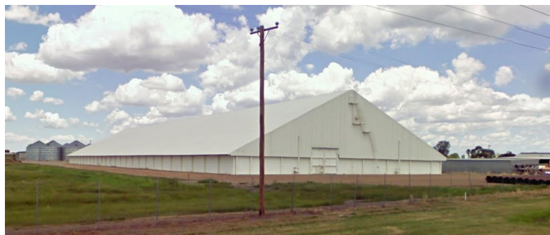
Figure 8: Typical grain storage and handling facility in Moree
