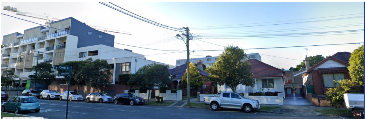
Rothschild and Queen, looking East. (left) 5 storey high density, (right) 1 storey res
