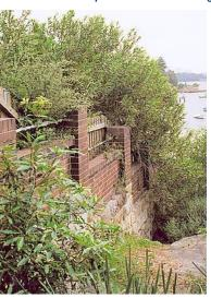
FIGURE 94 Composite wall containing sandstone and face brick on Salisbury Street
