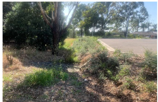
Figure 3 Vee Drain
